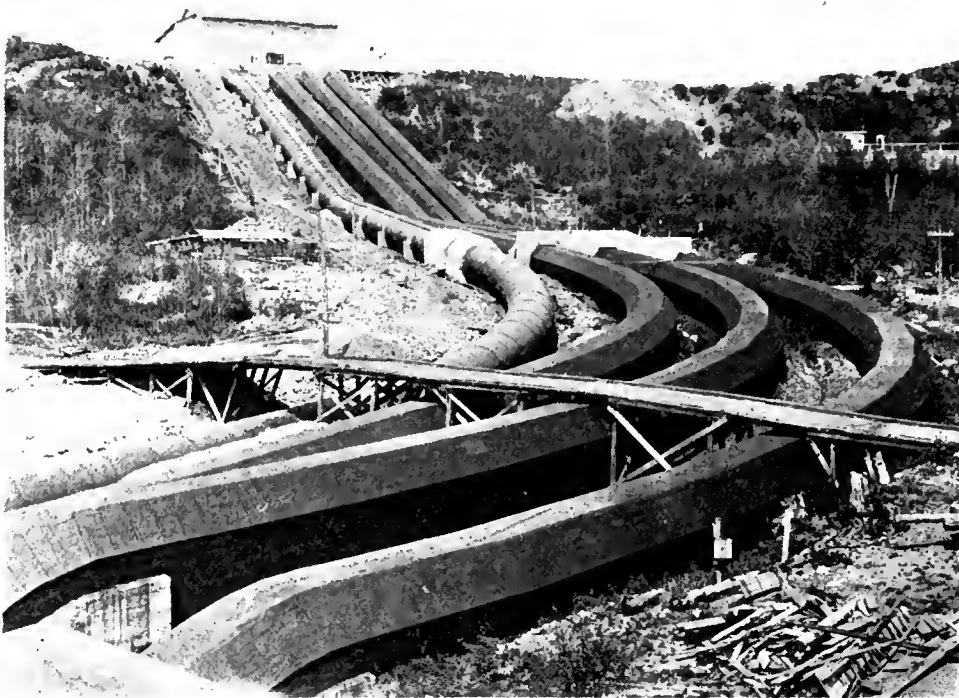
Forebay and Penstocks—No. 4, to left, 740 ft. long, 11 ft. diameter.
